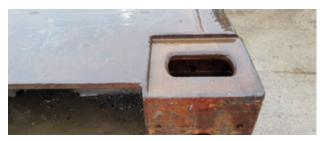
Chamfer on the lifting socket can be clearly seen.
